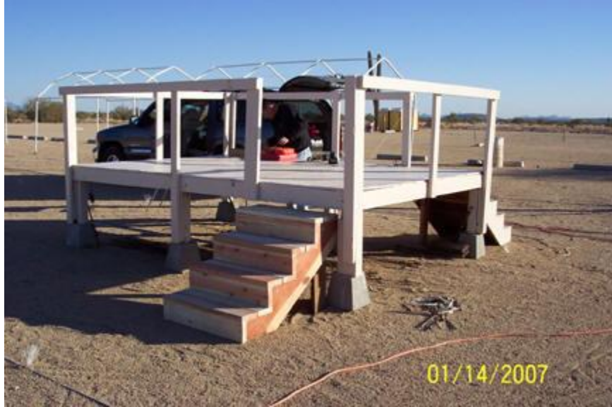
The second DOS stand stair has been built by Bob Pian.
